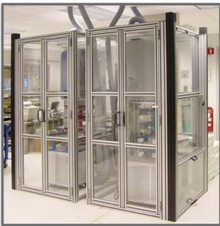
Walk-in hoods provide huge savings over dedicated rooms with special ventilation.
