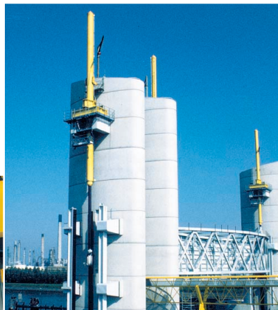
Ceramax cylinders for the Storm Surge Barrier in the Hartel canal at Rotterdam
