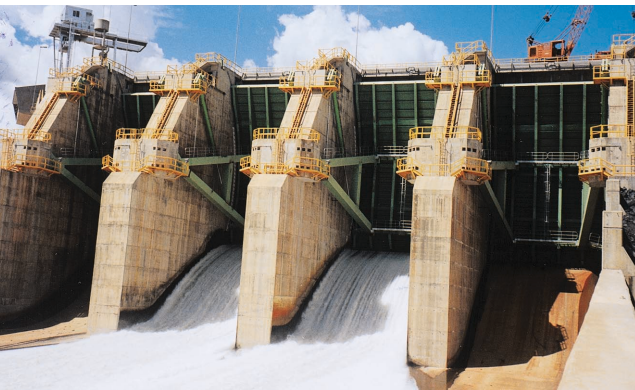
Miranda, Brazil equipped with ABS radial gate cylinders
